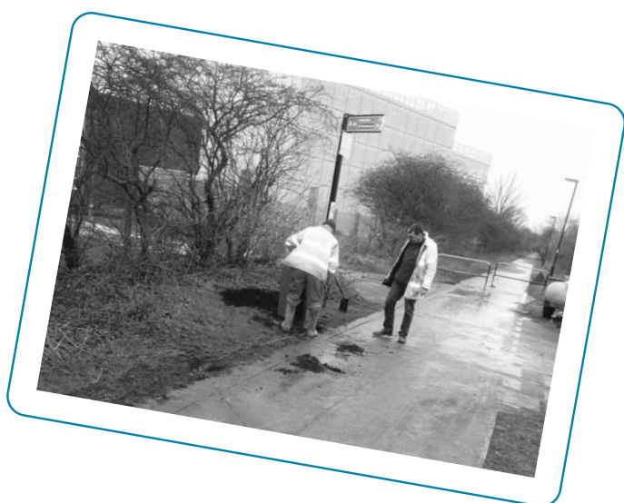
Cycling loop counters being installed on Coxlodge waggonway.
