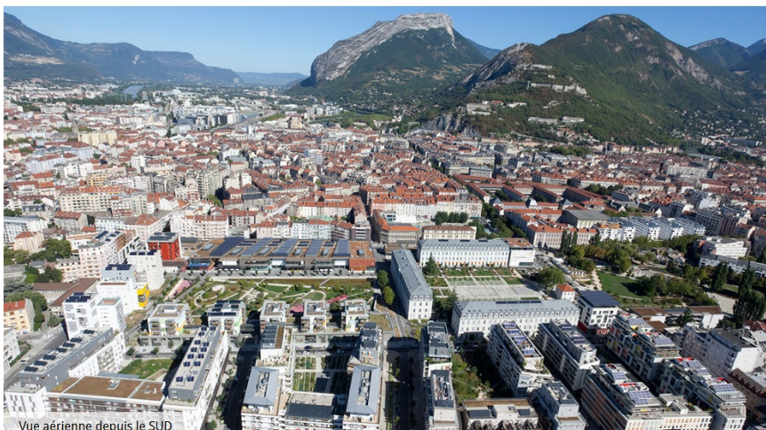
Source: City of Grenoble
